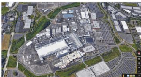
Typical industrial “supercampus”
